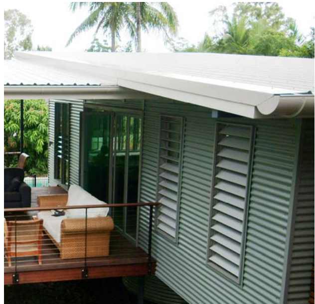
Aluminium louvres control western sun while allowing ventilation
